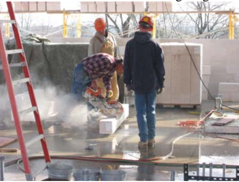
Field cutting lintel to length with chop saw
