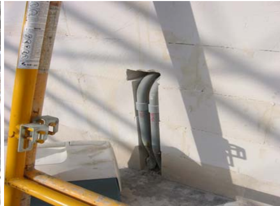
Flexibility of AAC Routed AAC block for electrical conduit run
