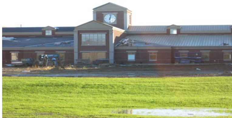
OSFC funded high school utilizes AAC cladding installed by Miles-McClellan Construction
