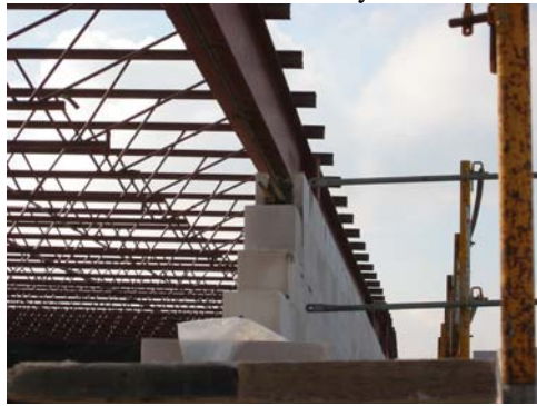
Ring beam intersecting with rafter beam
