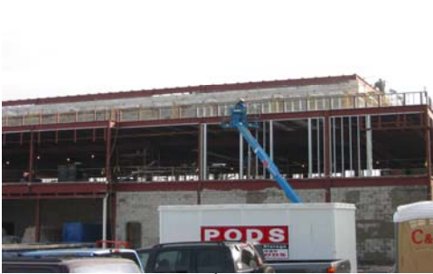
Ground view of 3 rd floor firing range
