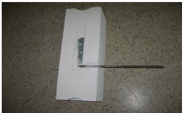
AAC block routed to accept threaded rod and flange.
